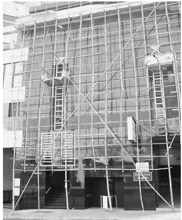
Fig. 1. Single Layered Bamboo Scaffolds (SLBS).
