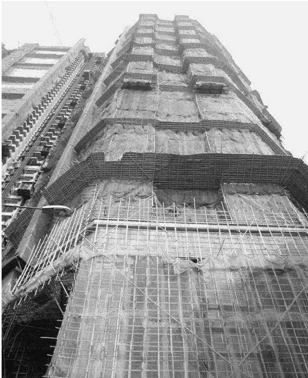
Fig. 2. Double Layered Bamboo Scaffolds (DLBS).
